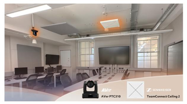
After extensive evaluation, Sennheiser's TeamConnect Ceiling 2 (TCC 2) microphone solution emerged as the most effective option. The microphone could also be integrated with the AVer cameras using the AVer PTZ Link software bridge so that both the camera and microphone could intelligently detect and follow the active speaker.
